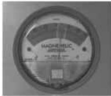
Image of room pressure gauge indicating colour coded normal, alert & action parameters
